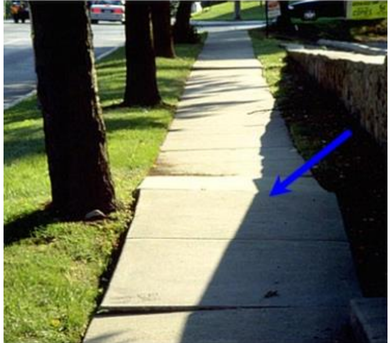
Figure G14. Ramping. Photo: Edward F. Gilman, Professor, Environmental Horticulture Department, IFAS, University of Florida
