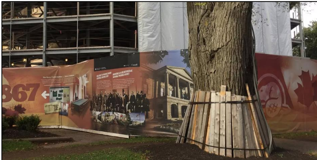
Figure 7: Example of tree trunk protection during construction. Source: National Park Service
