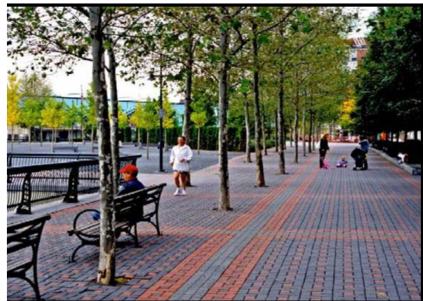
Figure G12. Permeable Pavers around trees, Hoboken, NJ Photo: Bruce Ferguson https://wiki.sustainabletechnologies.ca/wiki/Permeable_pavements
