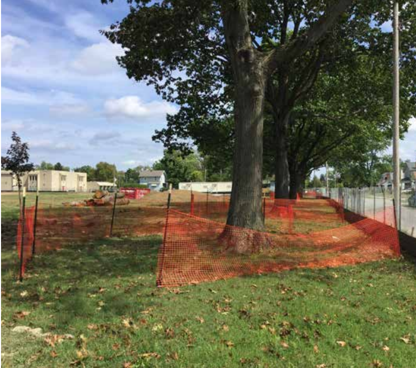
Figure 4.21 | Tree Protection Measures During Construction Tree protection fencing was critical to prevent damage to tree roots and subsequent tree loss during construction of Linden Park. ▲
